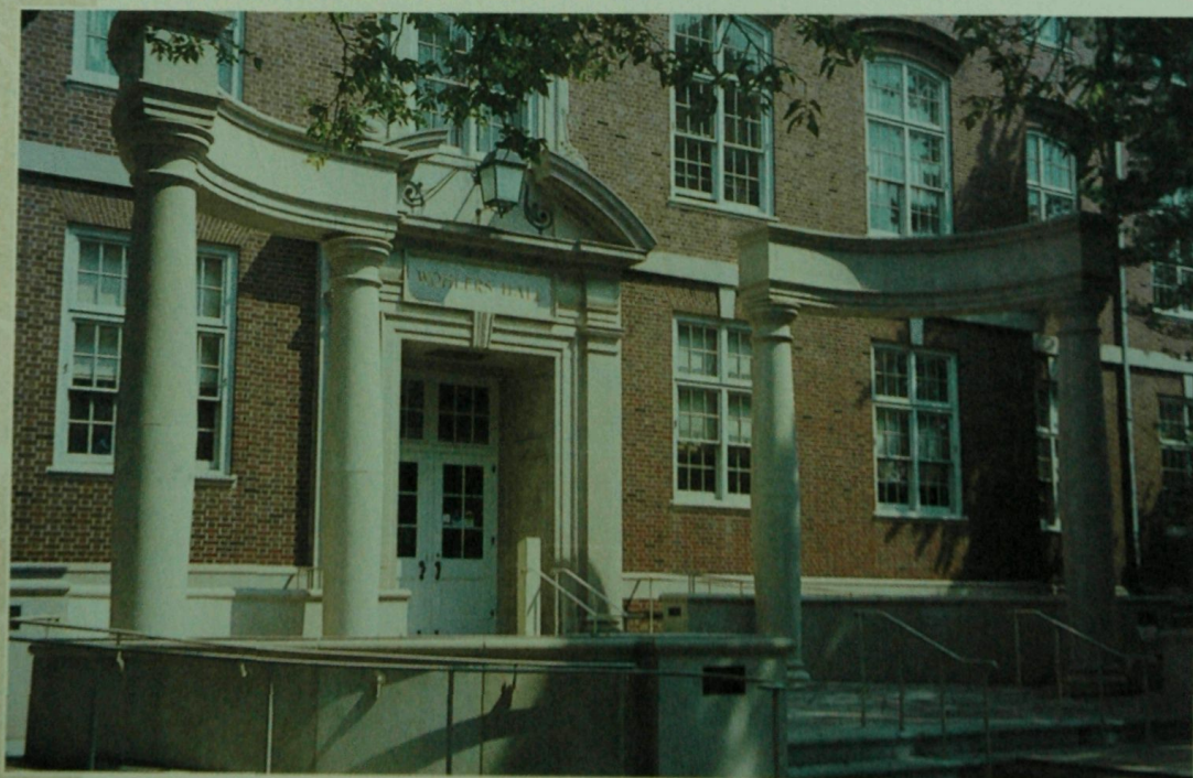
Central entrance to Woblers Hall
