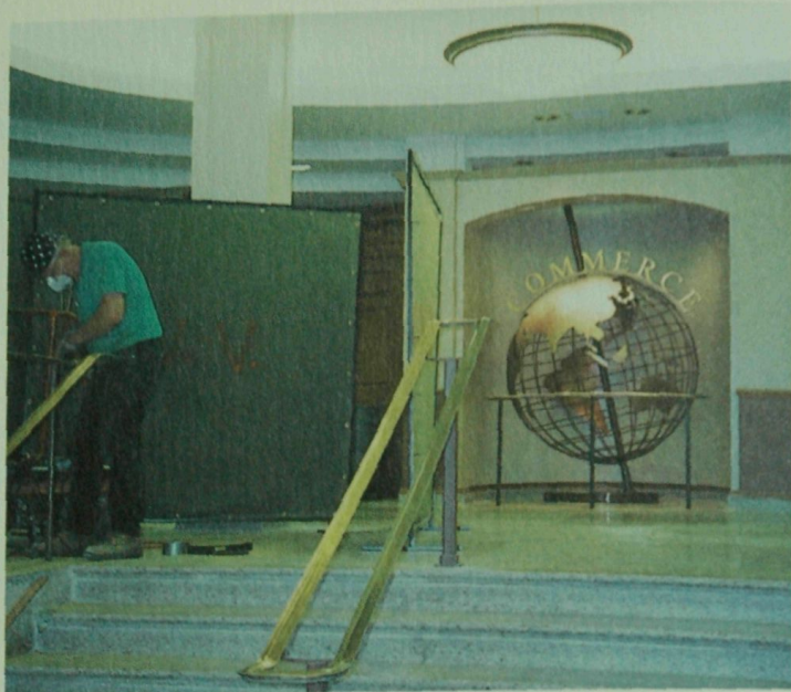
Putting the finishing touches on the new lobby
