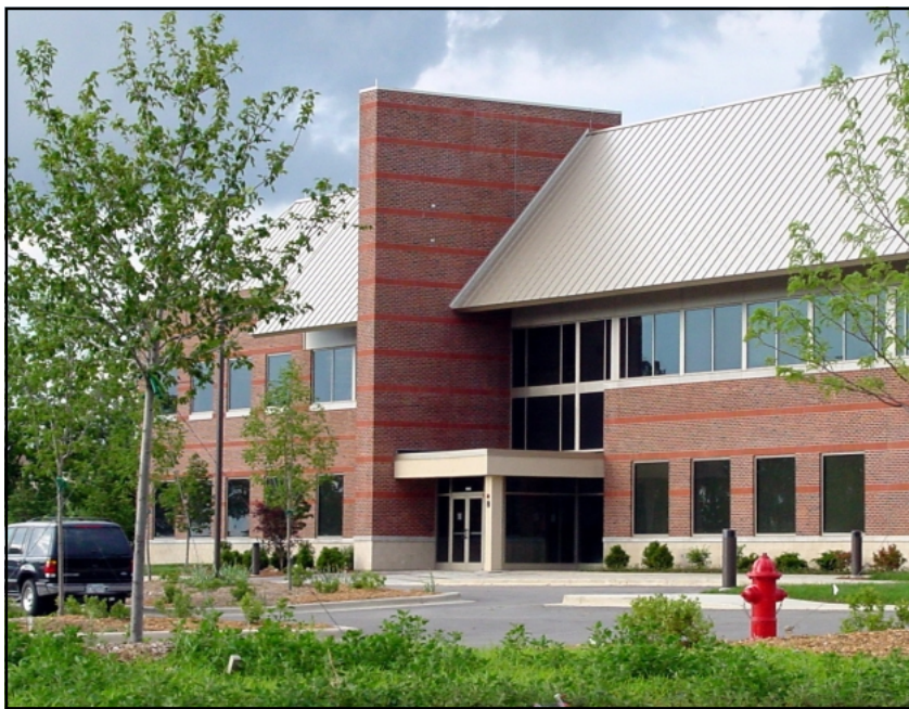
Fig. 18: Parking should follow the sequence Road-Parking-Building in an adequate balance with landscape.
