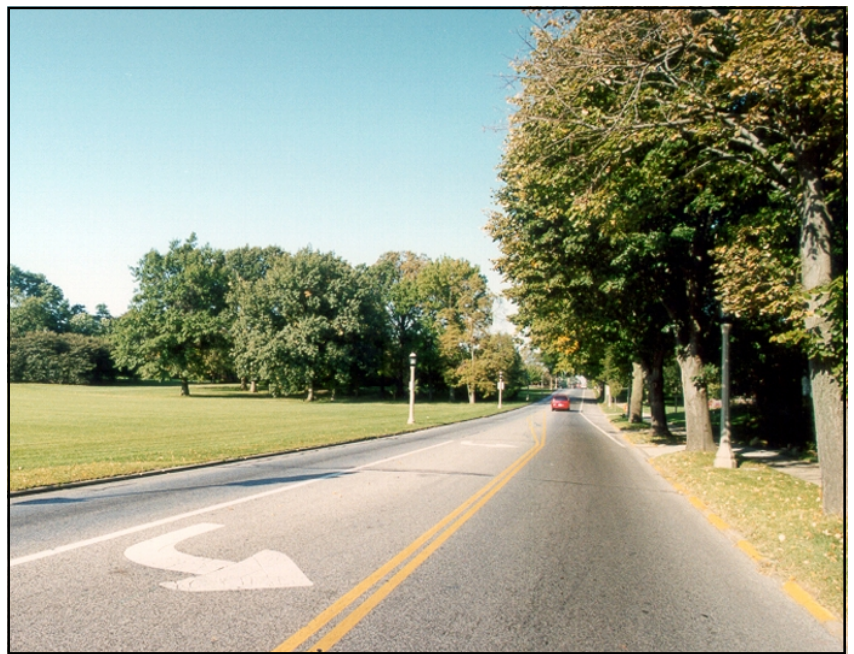
Fig. 16: The existing roadway system will be primarily maintained in its current location but upgraded to increase capacity.
