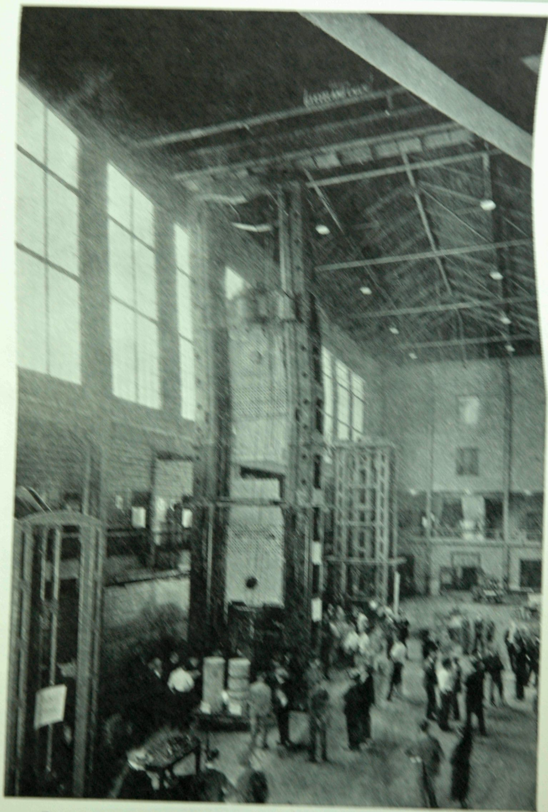
CRANE BAY, ARTHUR NEWELL TALBOT LABORATORY, SHOWING 3 000 000-POUND TESTING MACHINE IN OPERATION
