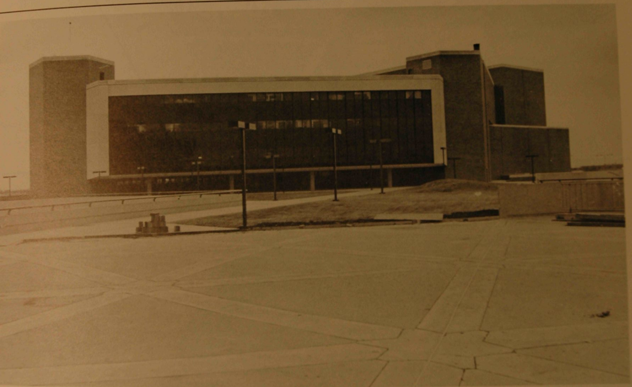
The completed PAC showing one of its glass faces
