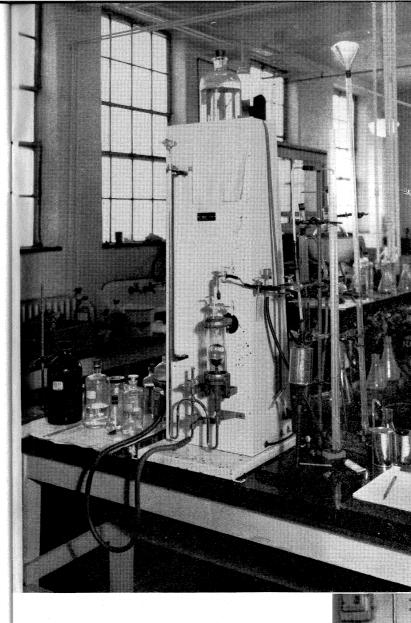
ONE of the studies being conducted by the Department of Food Technology has to do with the keeping quality of dried milk, cream and ice cream. The picture above shows the apparatus used to analyze the gas content of the air space in sealed containers of dried milk.
