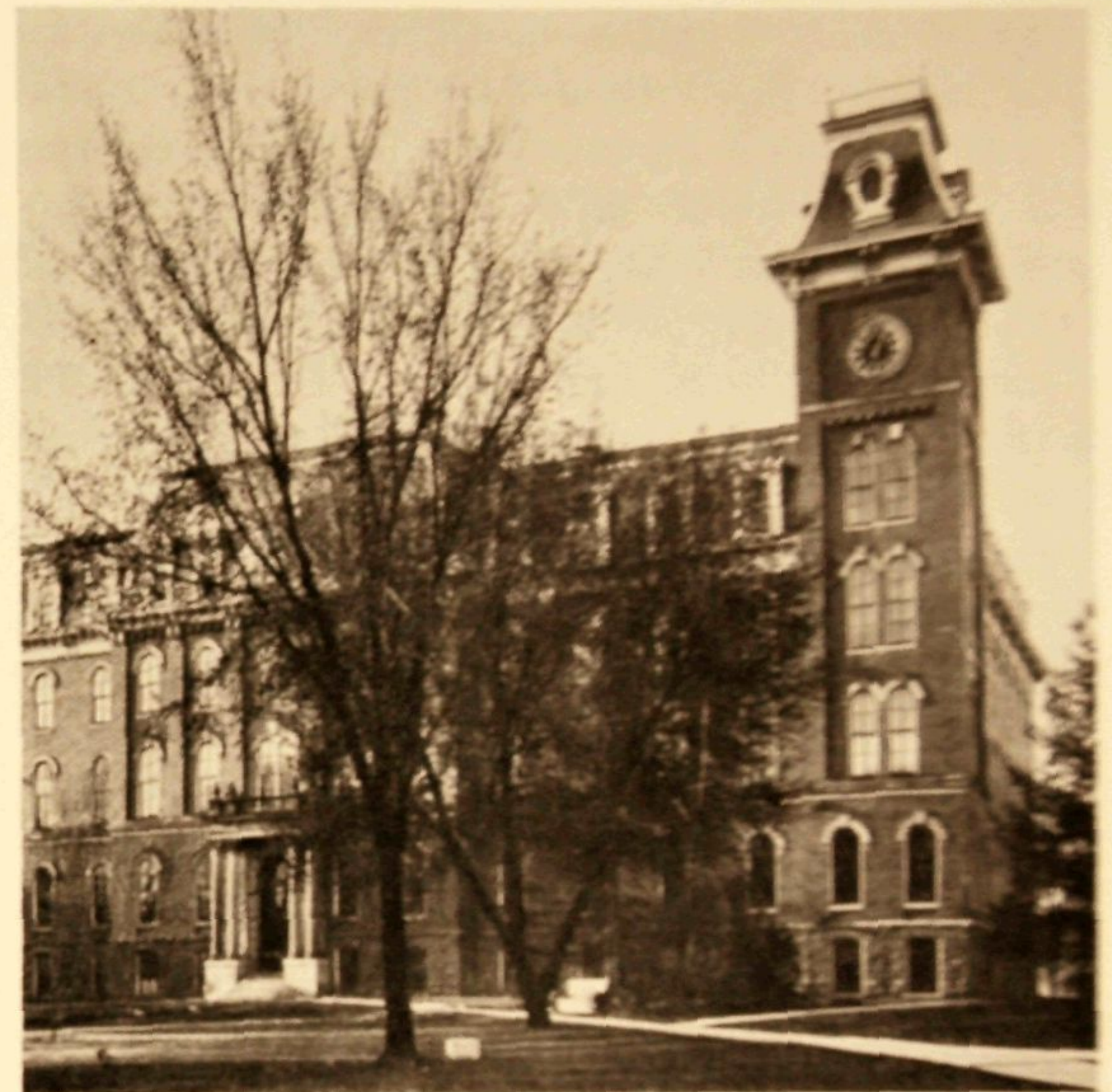
A COLLAPSED CEILING IN 1938 LED TO THE RAZING OF UNIVERSITY HALL, THE MAIN BUILDING FOR MANY YEARS.
