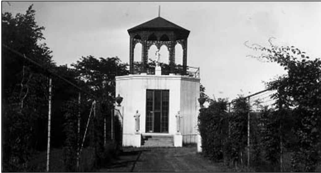
1925 (HGFF-03) Early view of the House of the Golden Buddhas with Vine Walk in foreground.
