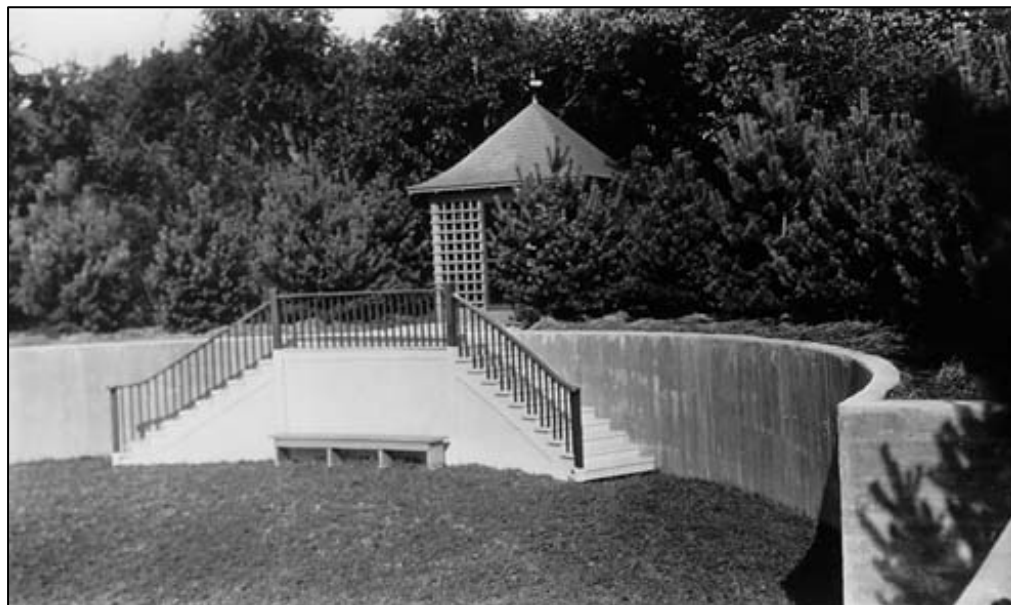
(HGS-3) Early detail of concrete stair and wooden gazebo. A two-story wood and concrete gazebo replaced this in the 1920s.
