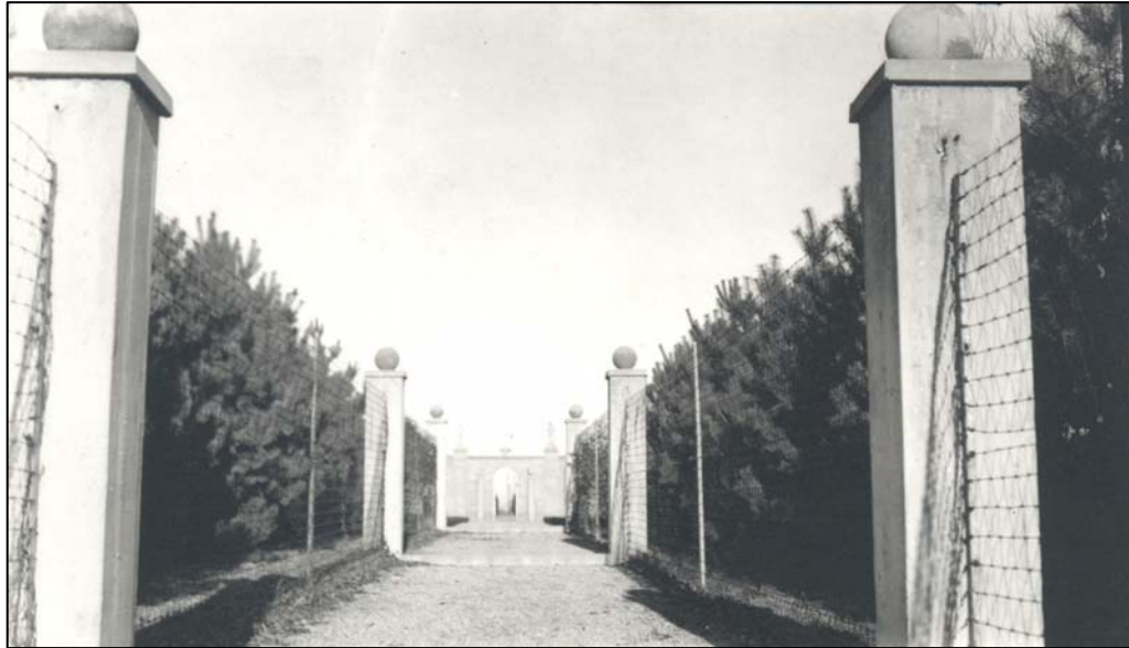
1912 (HGET-1) View east during construction circa 1912, with Chinese Maze Garden at rear. This garden was intended as an evergreen-lined passageway, punctuated by six pairs of columns surmounted by orbs. Wire trellises between the columns defined the edges of the space. This garden is lower in elevation than the Chinese Maze Garden, note steps at
