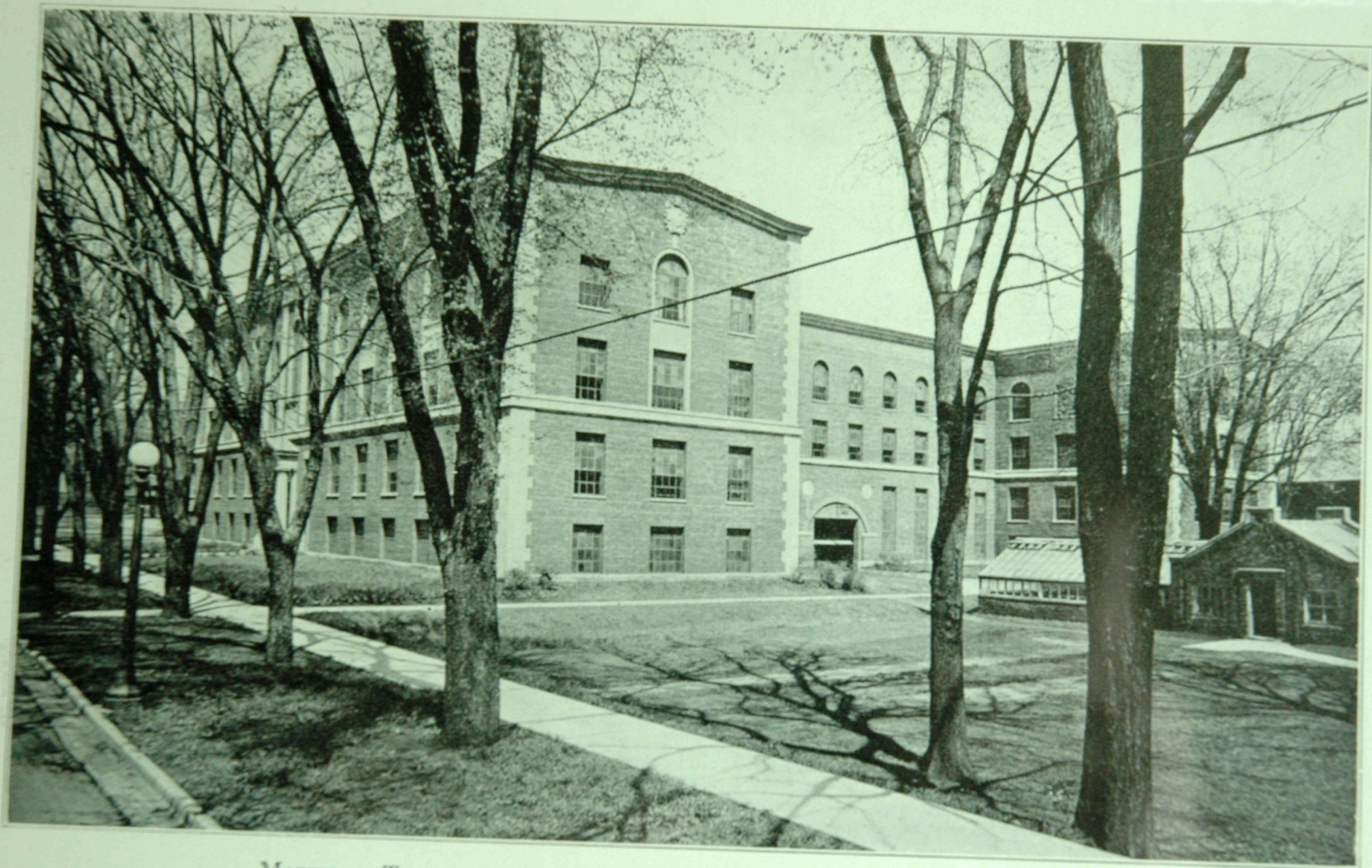
MATERIALS TESTING LABORATORY (LOOKING NORTHEAST FROM WRIGHT STREET)
