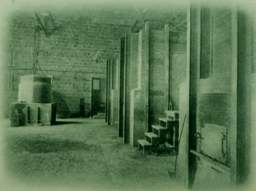
WEST END OF THE KILN LABORATORY SHOWING THREE COAL FIRED AND ONE OIL FIRED TEST KILNS
