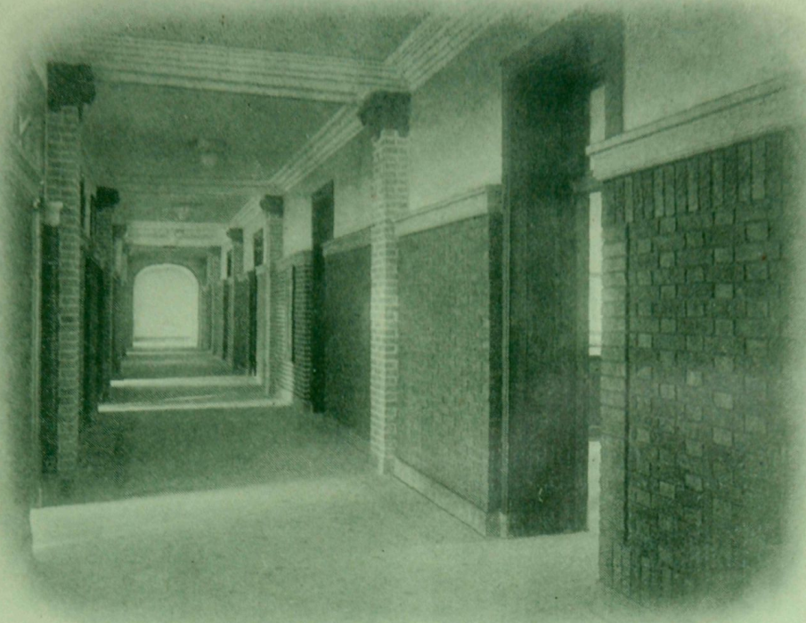
CORRIDOR ON THE FIRST FLOOR SHOWING DISPLAY PANELS OF DIFFERENT STYLES OF FACE BRICK
