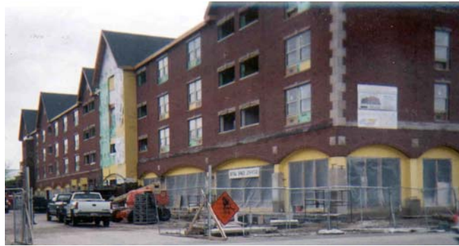
East Campus Commercial Area
