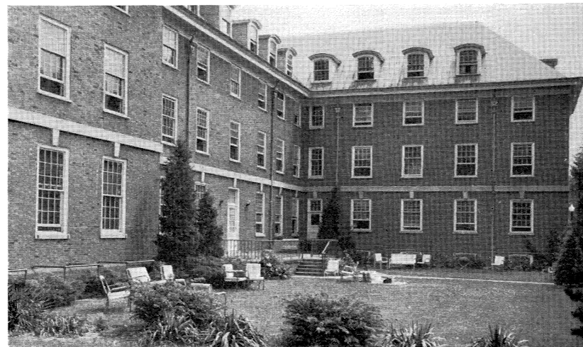
Back Terrace of One of the Women's Residence Halls
