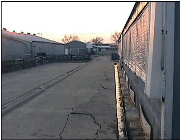
Existing Swine Facility ▲
