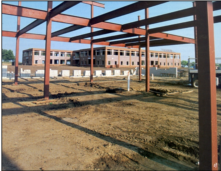
South Research Park Building under construction ▲
