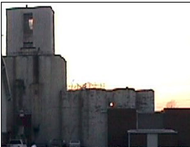
Existing Feed Mill ▲
