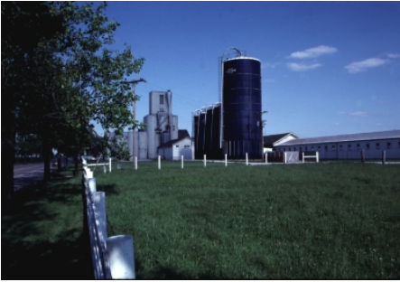
Obsolete Facilities along St. Mary's Road need to be replaced.
