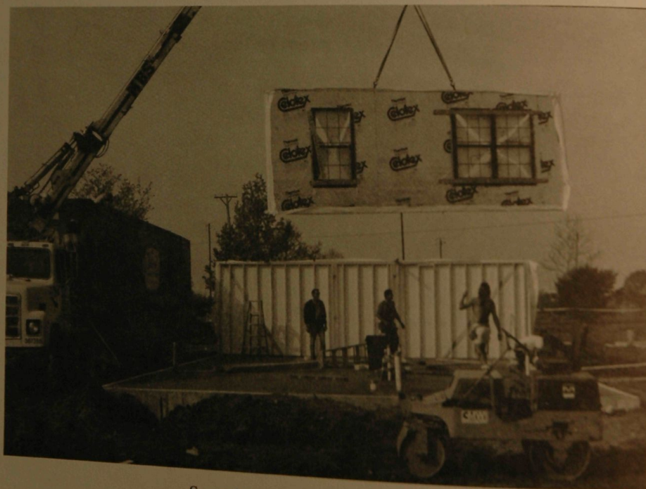
Second phase of student housing. Panelized housing units being erected – April 1990.
