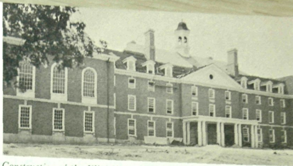
Construction of the Illini Union began in 1939.
