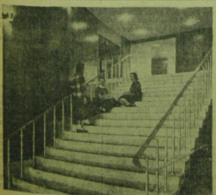
A wide stairway at the front entrance of Bevier Hall leads the way to the second floor student lounge. Striped panels of zebra wood extend from the first to the second floors in this entranceway and encase the stairway.
