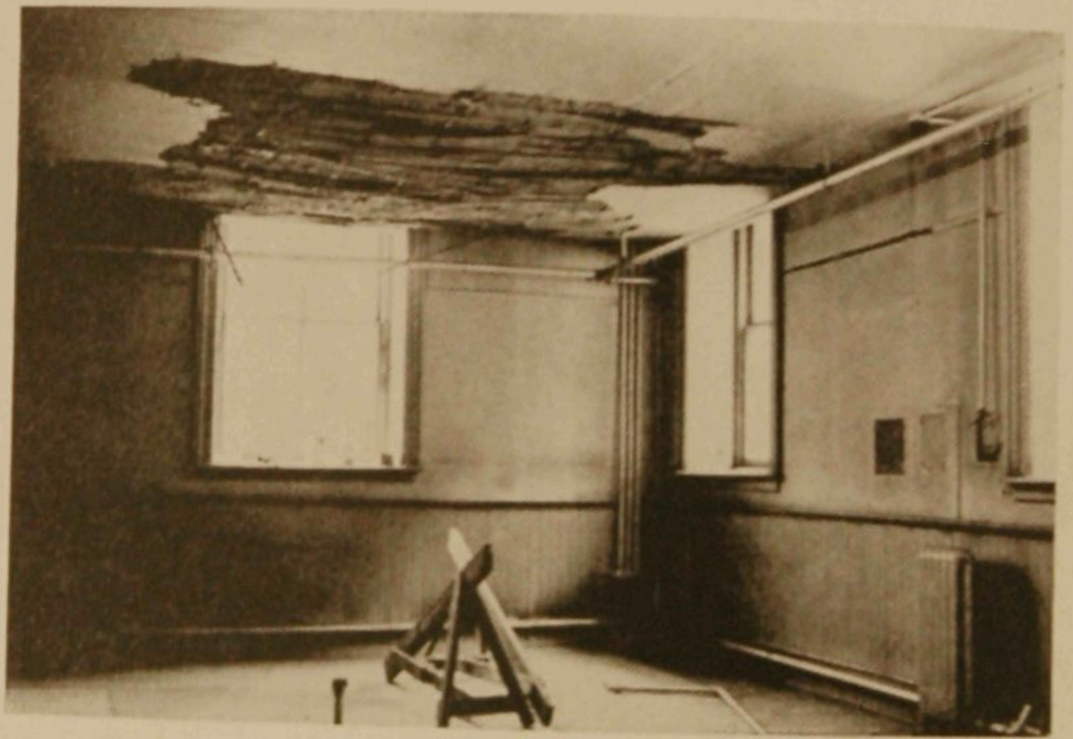
When the ceiling in University Hall collapsed, causing the building to be condemned, alumni mourned the razing.
