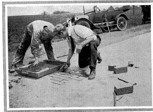
REPAIR ON BRICK ROAD
