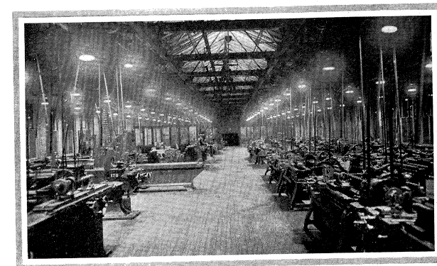
INTERIOR VIEW OF THE MACHINE SHOP
